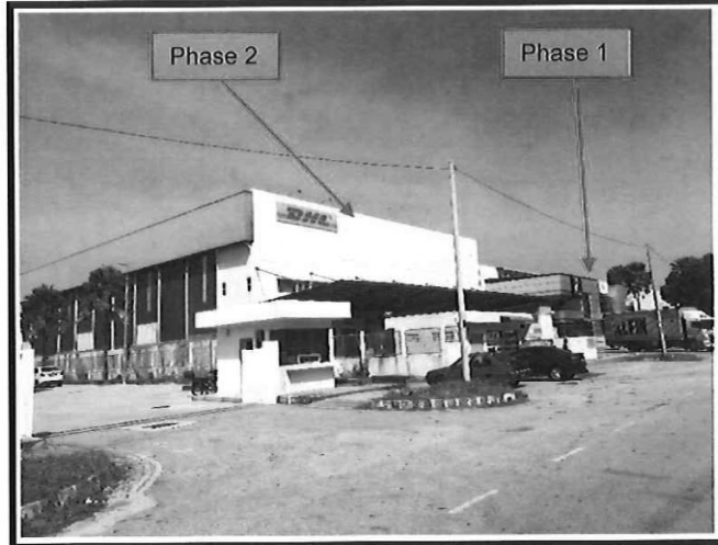
GENERAL VIEW OF SUBJECT PROPERTY
